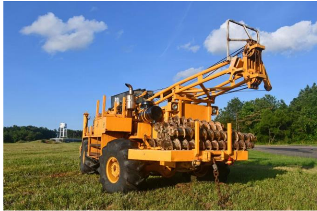
Site Preparation Equipment Lake Martin Regional Industrial Park, Kellyton, AL
